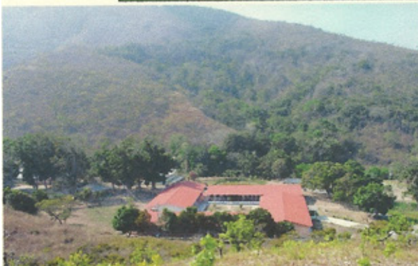
Beginnings. March 21, 2001. SAH buildings,
